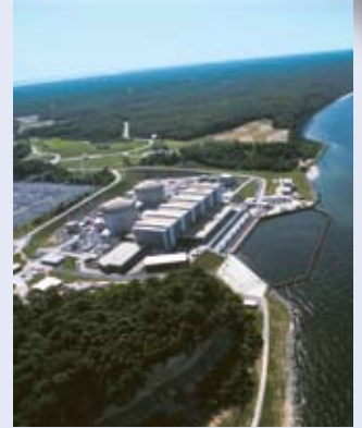
Calvert Cliffs Nuclear Power Plant, Lusby, Md.
